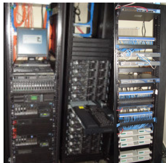
P-series Servers 42 U Rack X-series Servers 42U Rack Networking components 45U Rack
